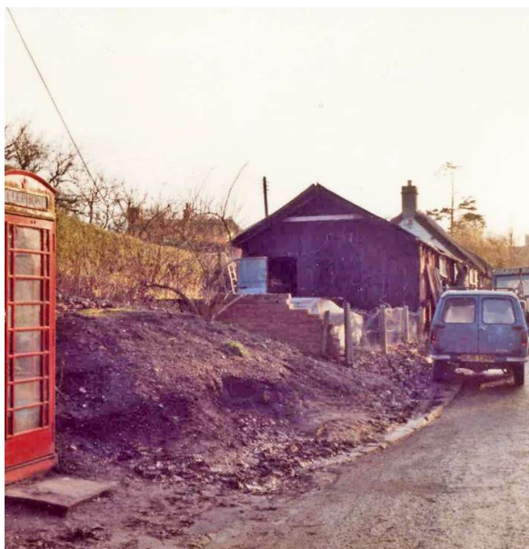
The Old Rifle Range before reconstruction began.
