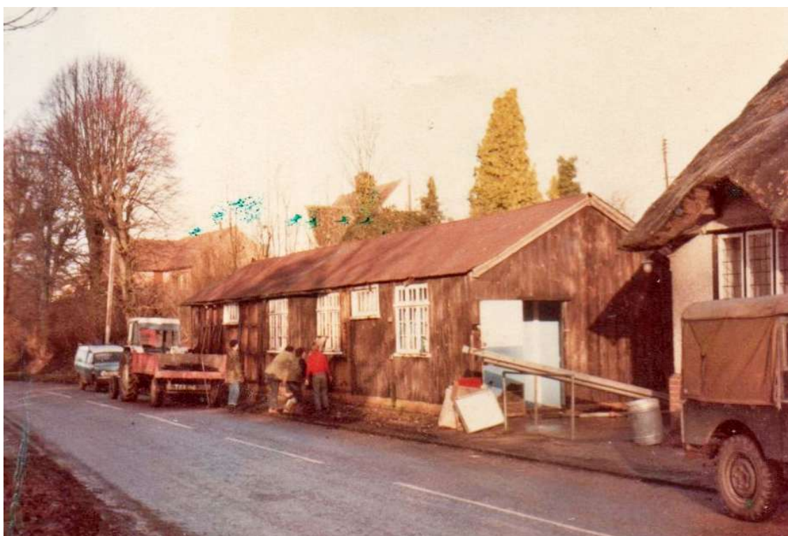
The Old Rifle Range before reconstruction began.
