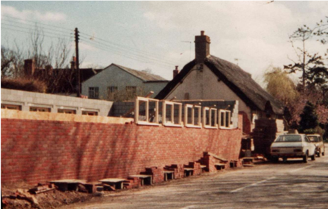
The building of the new Village Hall commences.
