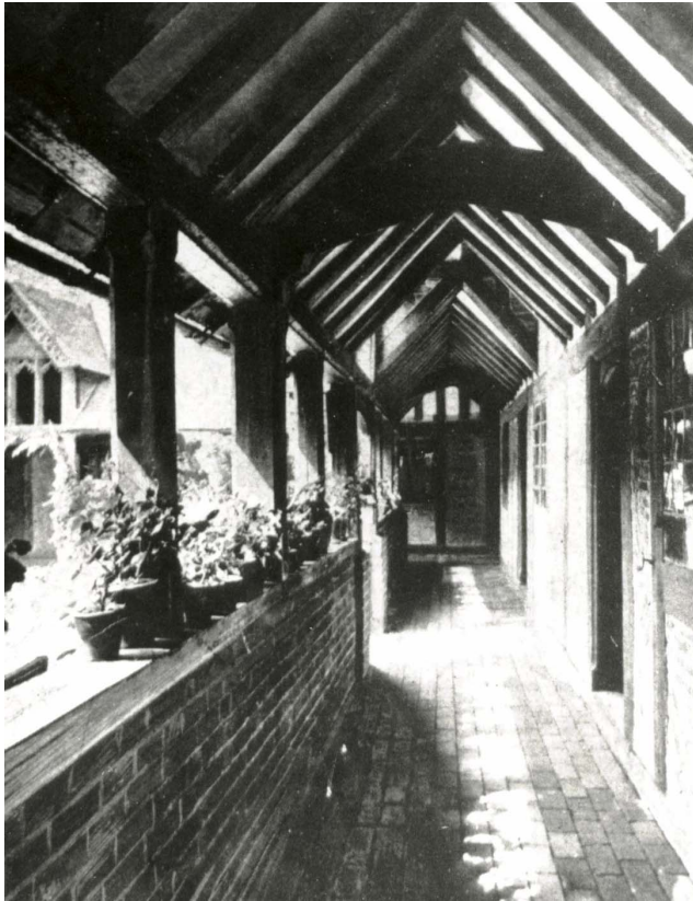
The Cloisters Ewelme Almshouses
