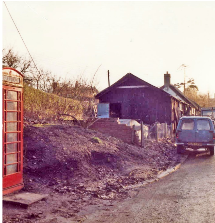
Demolition of the old building.
