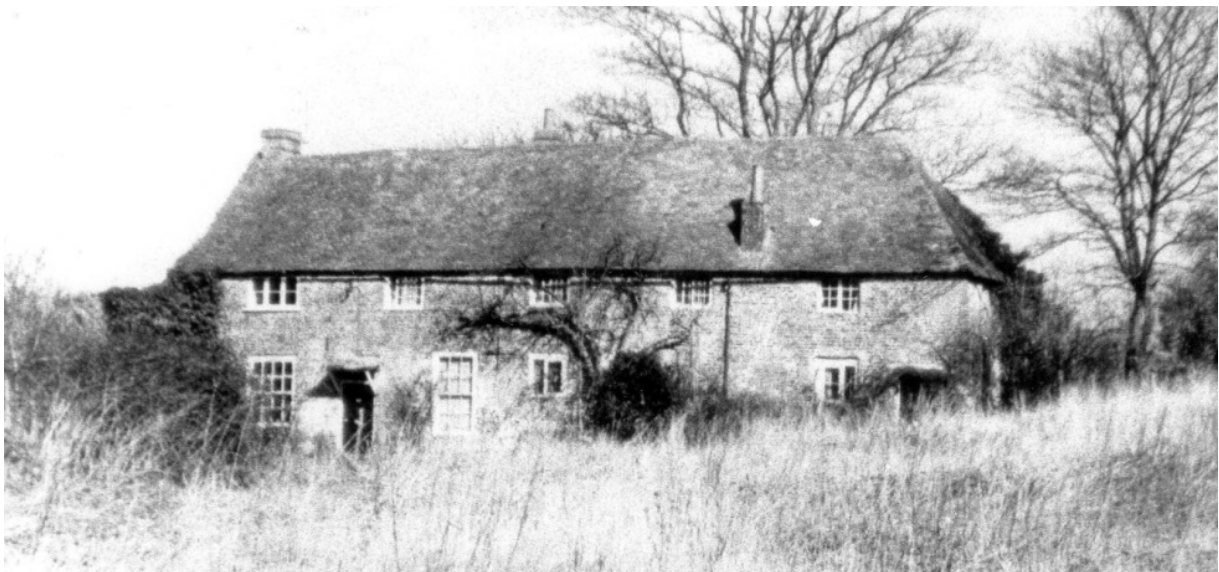
The Mount shortly before demolition
