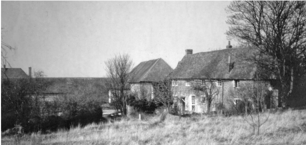
The Mount shortly before demolition
