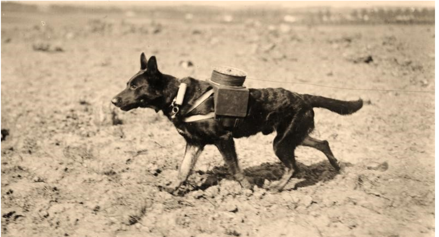
Laying a telephone wire.
